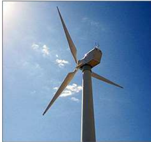
Northern Power Systems 100-kW wind turbine
