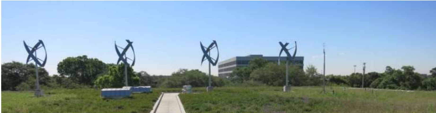
NASA Building 12 wind turbine installations. Photo by Dave Jager, NREL
