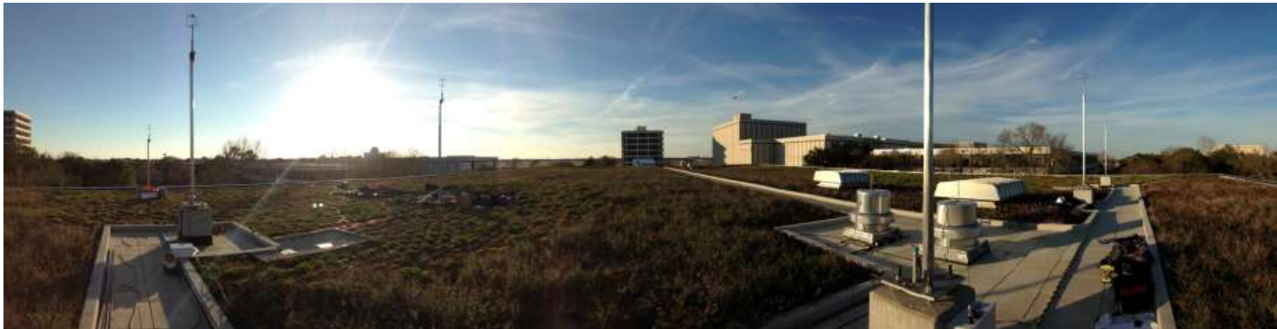
NASA Building 12, Phase 1. Photo from Jason Fields, National Renewable Energy Laboratory
