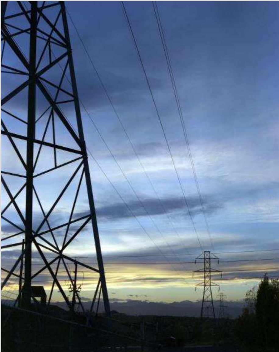
Photo by Warren Gretz, NREL 00002
