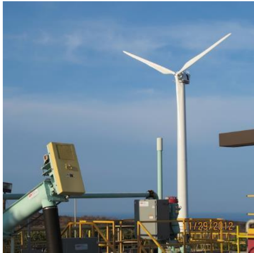
Northern Power Systems 100-kw wind turbine, Photo by Northern Power Systems, NREL 26787
